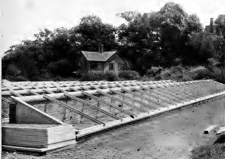
Coldframes of brick and iron
